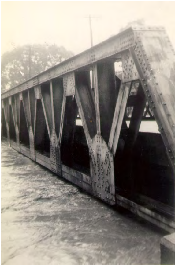
Five Mile Creek Bridge - Rt. 17
