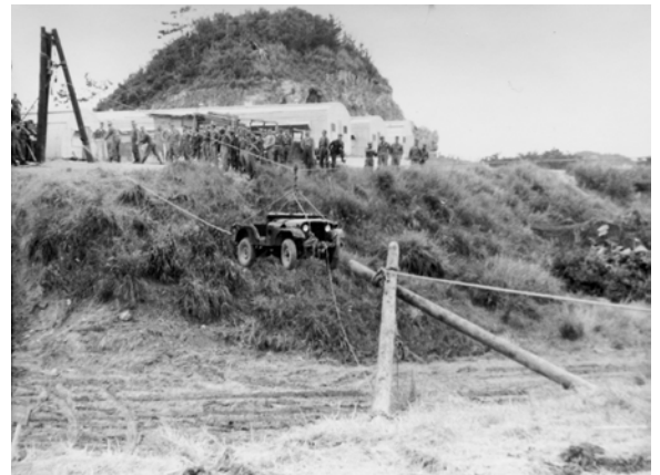
Training - Cabling M151 Across Ravine
